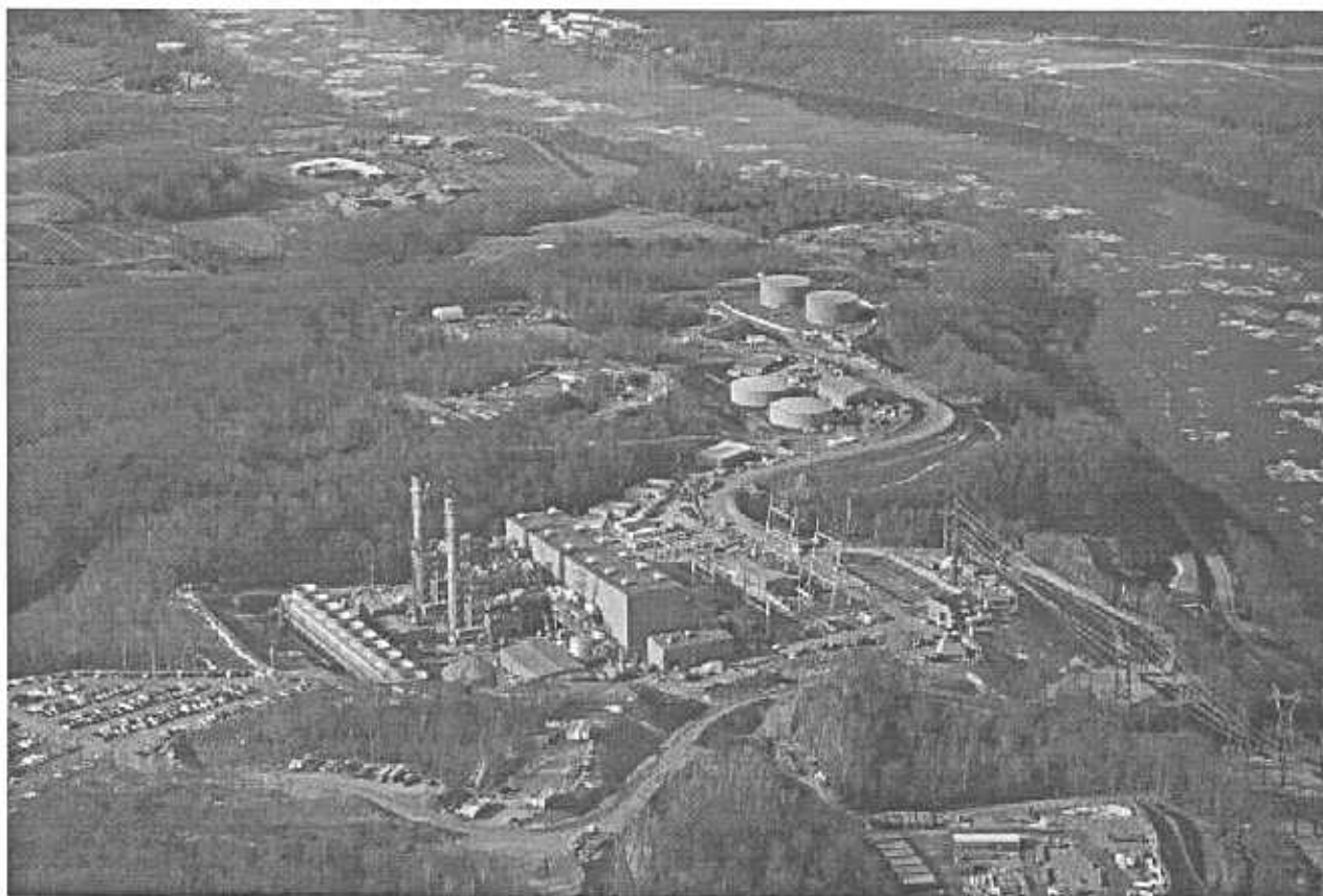
Power Block Overview
